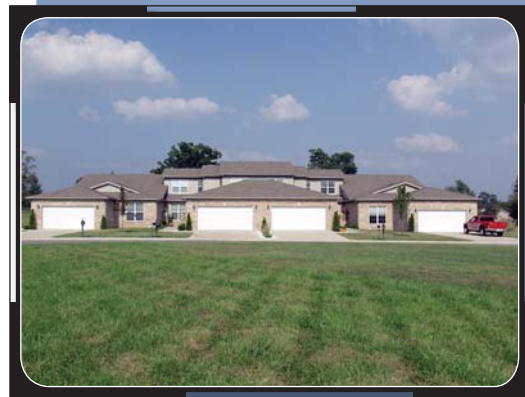
Drip field location
